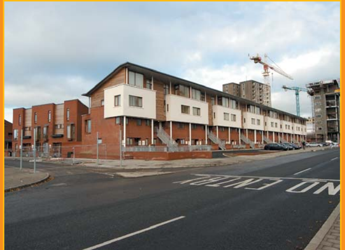
Gateway housing almost complete
