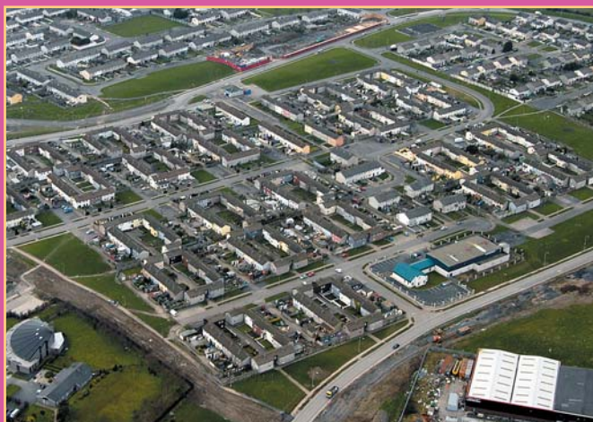
Aerial view of courts
