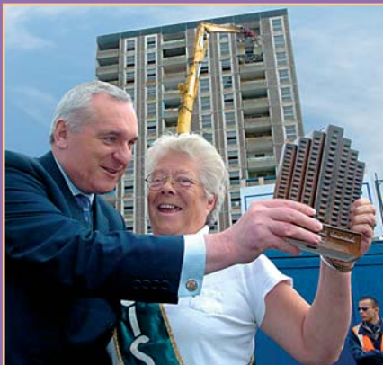
An Taoiseach Bertie Ahern and Queeny Barnes at the Demolition Ceremony on Saturday 10th July 2004.
