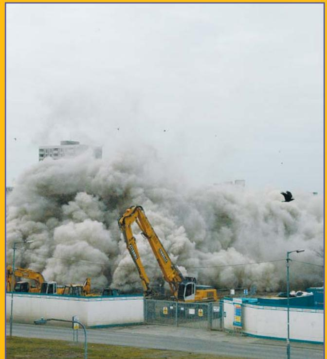
MacDermott Tower was the seventh block of Ballymun flats to be demolished and the first to be demolished by explosives. The highly successful operation was choreographed with meticulous timing by Tinnelly Demolition. Pearse Tower was demolished in July 2004, while McDonagh and Ceannt Towers are currently being slowly demolished by mechanical means.
