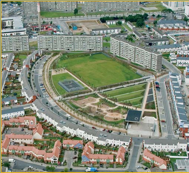
The new Coultry Park
