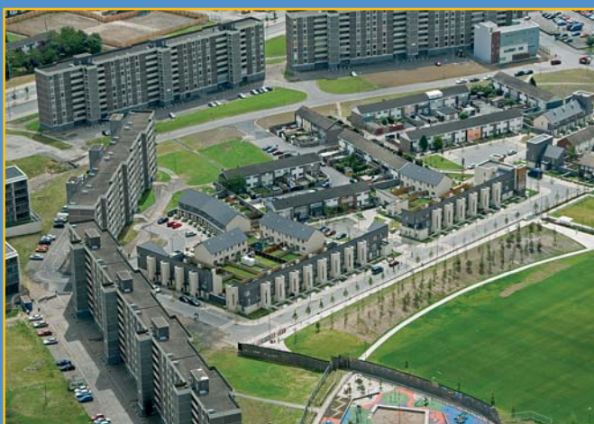
Balbutcher 1 which was recently completed and is now occupied
