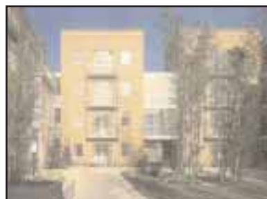
Private Rented Accommodation U.K.
